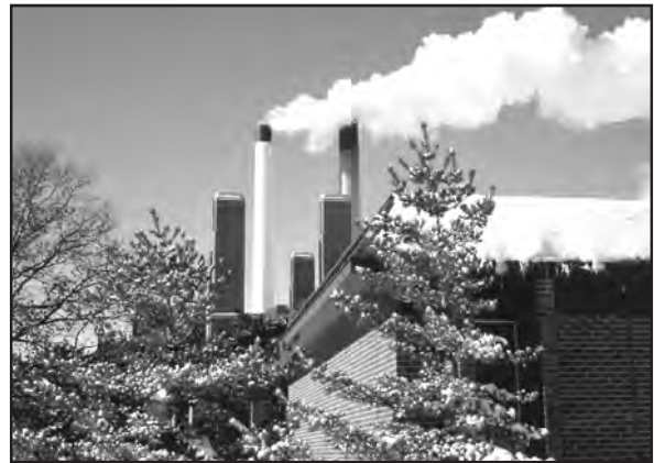
Coal-powered Abbott Power Plant, Champaign, Illinois.
